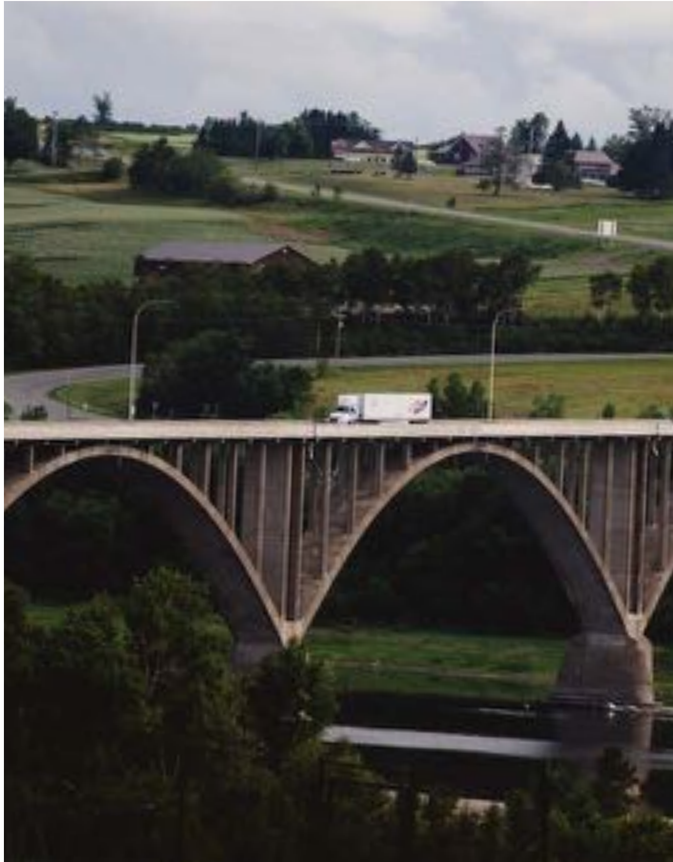
Hugh John Flemming Bridge, Hartland, New Brunswick
